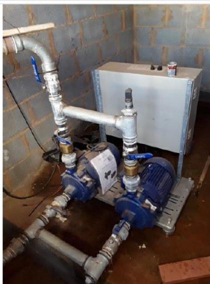
Painel de controle
